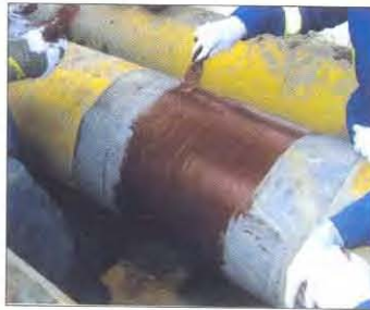
Apply 2-part Epoxy/#Z704 Rustex
