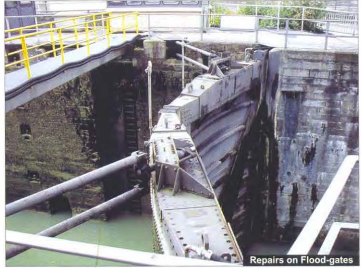
Repairs on Flood-gates
