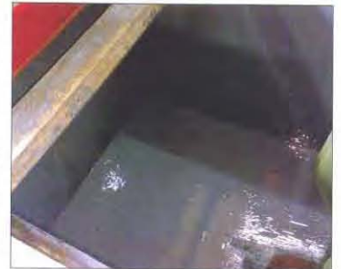
Coating in LRS Tank
