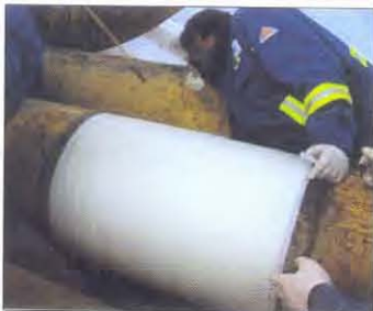
30 Minutes later, project complete
