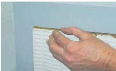
4.) ... and put into the opening (coated side = outer side).
