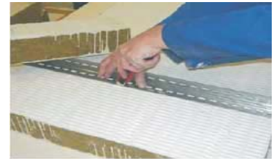
3.) Pre-coated firestop board A150 is cut to required size ...
