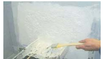
6.) Complete the installation coating with "A107" (depth of layer approx. 1-2mm) and also cover the joints and gaps.
