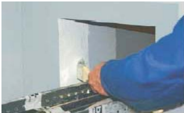
1.) Cleaning of opening, put adhesive tape around it to obtain an even rim (50mm), apply "A77" on inner side of opening ...
